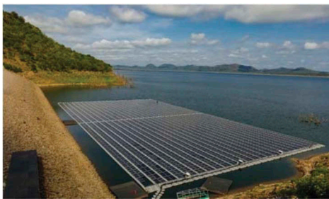
Figure 11. One MW floating solar at Bui, Bono East Region (Ghana) (Power Africa 2022).
